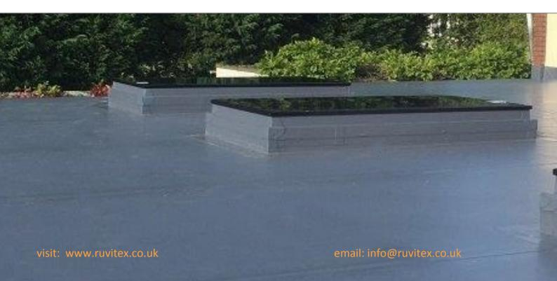
Ruvitex Mechanically Fixed Overlap System is suitable for warm roof constructions incorporating thermal insulation as well as cold roof and renovation projects.
